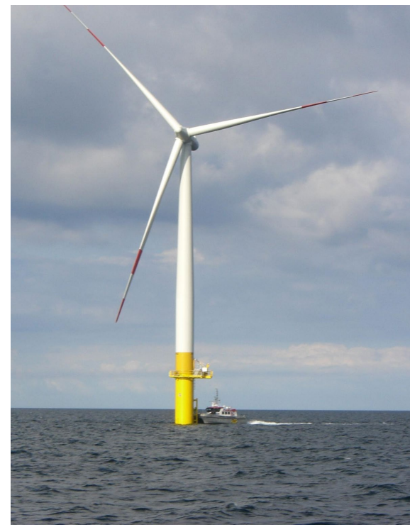
Baltic-1 2.3-MW Siemens fixed-bottom wind turbine in Germany; 2010 monopile substructure. Photo by Walt Musial
