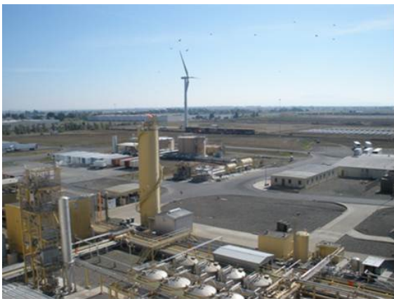
A 1.5-MW GE wind turbine at Anheuser-Busch in Fairfield, California, provide 25% of facility's load. Photo from Foundation Windpower, NREL 26500.
