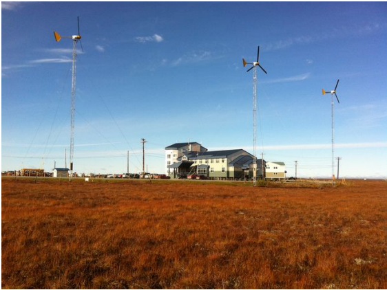
Three Excel 10S turbines on 80-foot GL towers provide power to a school in Bethel, Alaska. Photo from Pieter Huebner, NREL 26471
