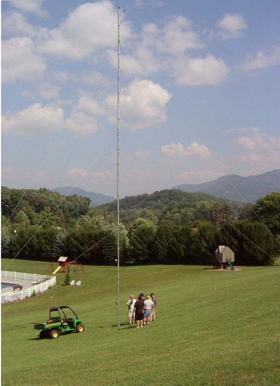
A team from Appalachian State University installs a wind measurement tower. Photo from Appalachian State University, NREL 15302
