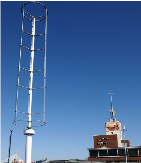
A vertical access wind turbine installed at the Boston Museum of Science. Photo from Boston Museum of Science
