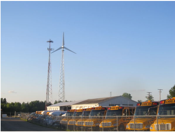
Myers Equipment Corp. - a full-service distributor of school buses, ambulances, and other truck equipment - is powered in part by a 50-kilowatt wind turbine. Photo from United Wind , NREL 26772
