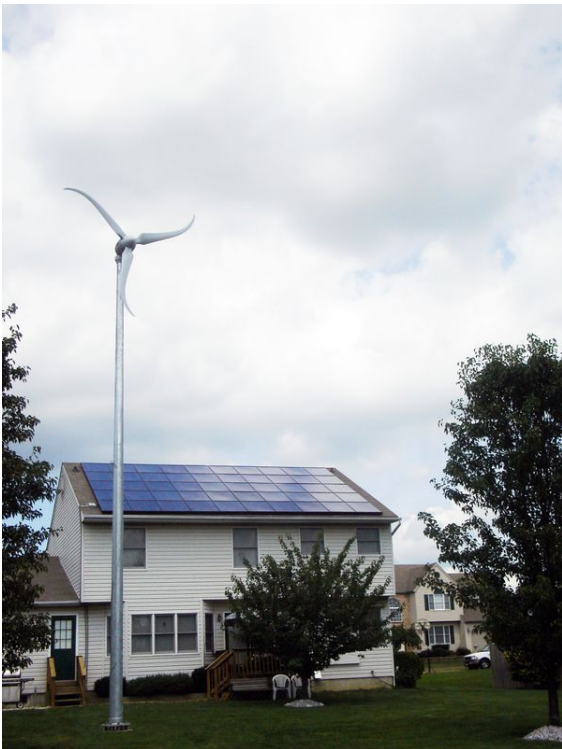
A Skystream turbine in a residential application. Photo from Southwest Windpower
