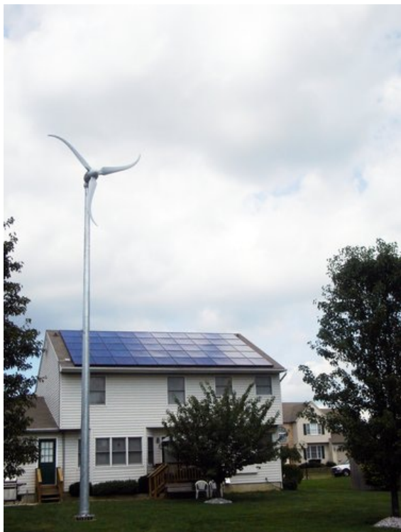
Southwest Windpower's 1.8-kW Skystream wind turbine in a residential application. Photo from Southwest Windpower, NREL 14936
