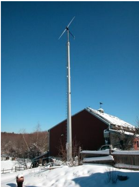
This Southwest Windpower Whisper 175 wind turbine on the Lion Spring Farm in Dover, Massachusetts, supplies electricity for the house and barn. Photo from Bob Michelson Photography, NREL 12564
