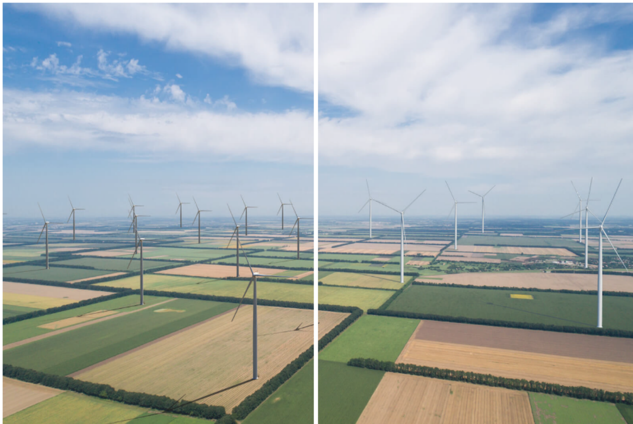
Figure 9 (left) and 10. These images highlight the potential changes that can occur during a full repower of a wind energy project. Older, smaller wind turbines (left) can be replaced with fewer, newer, larger models that could have the same total capacity (right). Images by Josh Bauer, NREL
