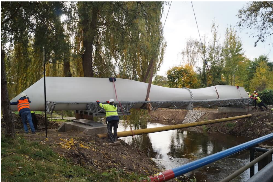
Figure 1. Construction workers install a footbridge across the Szprotawa River in Poland. The footbridge was designed and constructed by Anmet, a Polish recycling company, whose designs feature repurposed wind turbine blades. Photo from Anmet.
