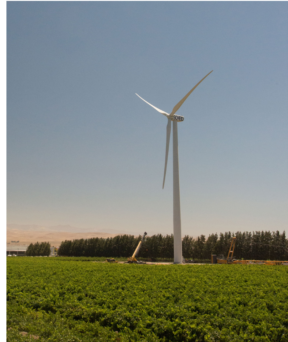
This 1.85-MW GE wind turbine powers an industrial vineyard operation in California.
