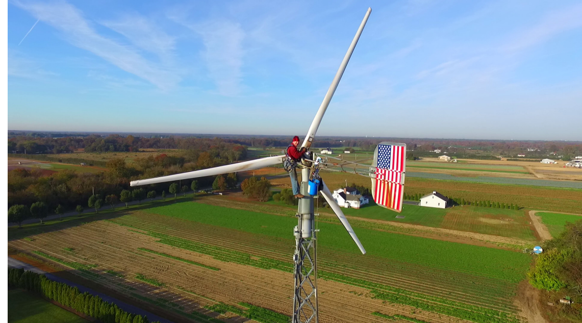
A maintenance provider servicing a 20-kW Jacobs 31-20 wind turbine on a farm. Photo Credit: Roger Dixon / Skylands Renewable Energy LLC
