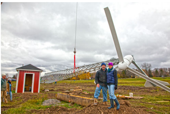
A Bergey 10-kW turbine being installed on a 120' SSL tower for a winery in Lockport, New York. Credit: Niagara Wind & Solar, Inc.
